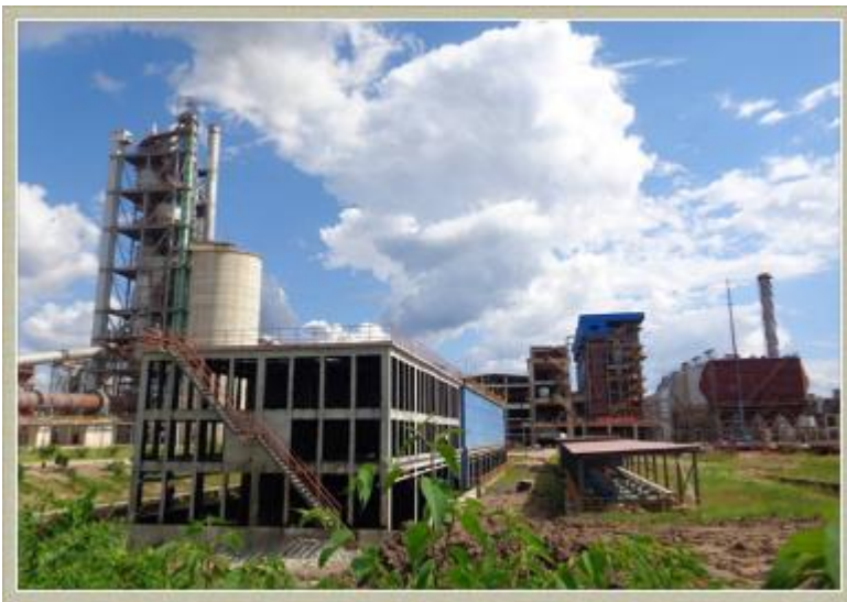
The full view of Captive power plant in Muara Satui ,Indonesia
