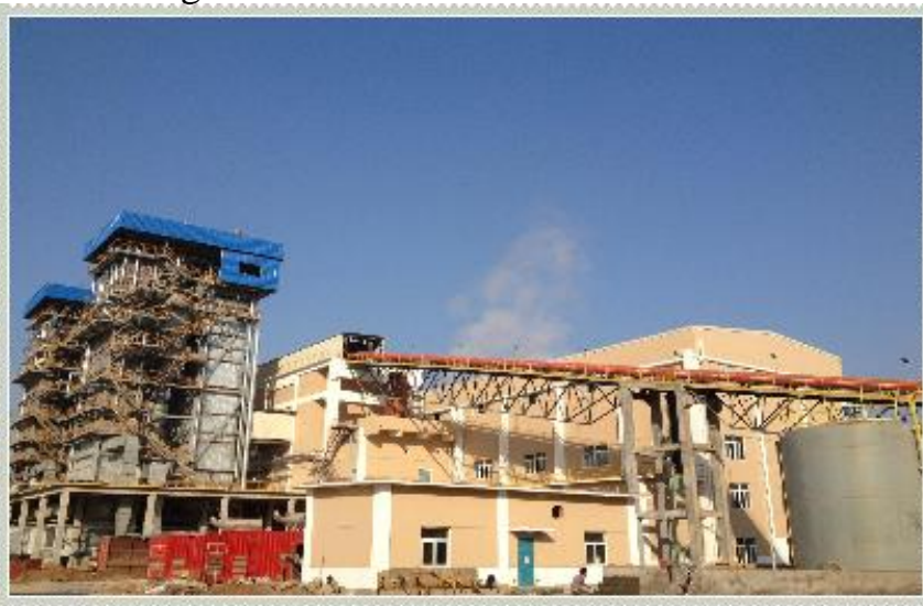
The Coal Fired Power Plant built by Company in Kyaukse, Myanmar
