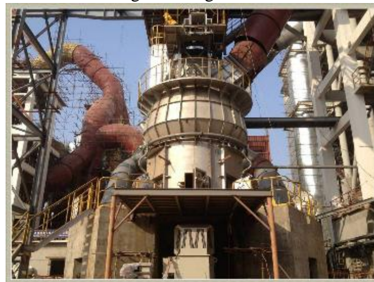
Vertical Mills Project in Kyaukse, Myanmar
