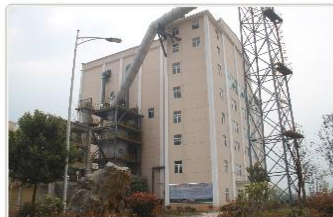
Plant area of garbage disposal project in Qiyang, Hunan Province
