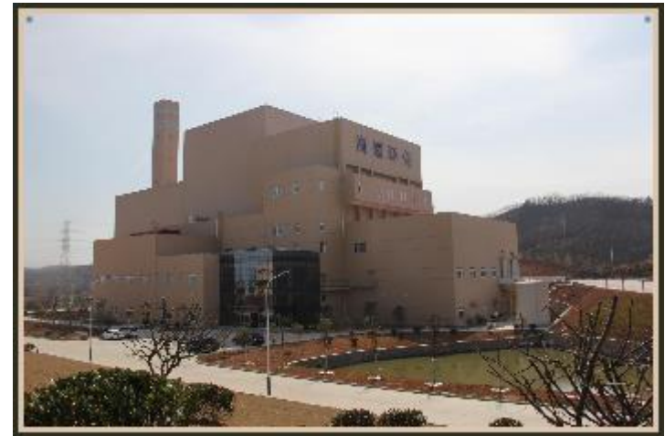
Grate furnace in Jinzhai of Anhui Province was put into operation at the end of 2015.
